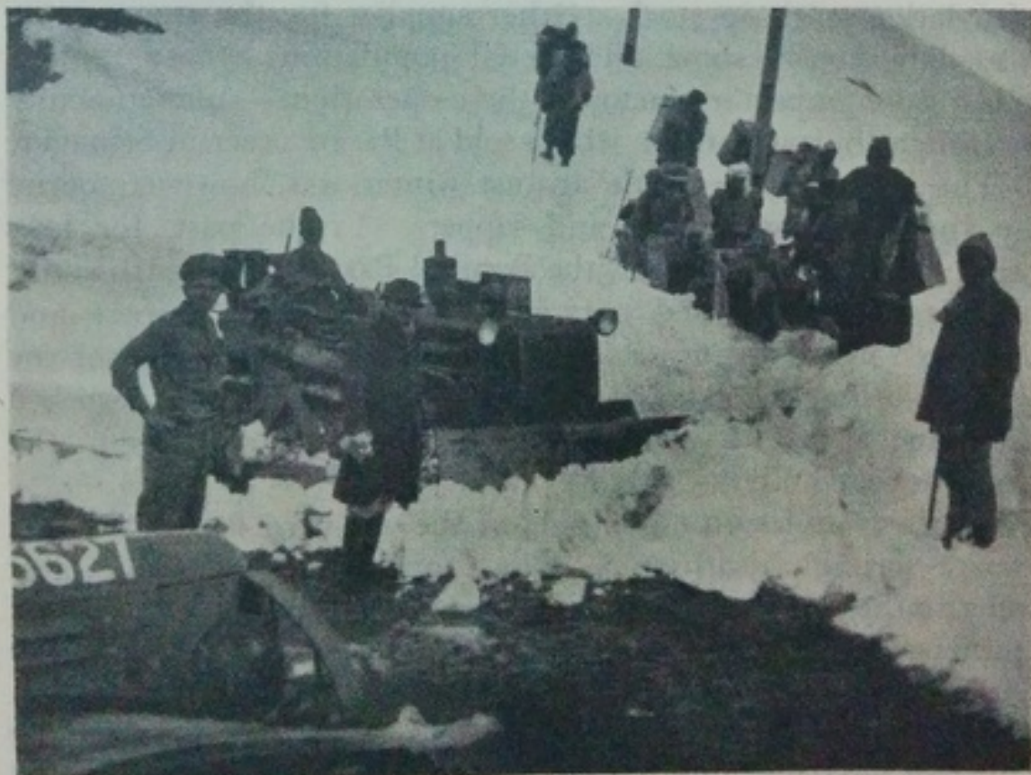
A bull-dozer clearing the snow on the Banihal Pass at a height of over 9,000 ft.
